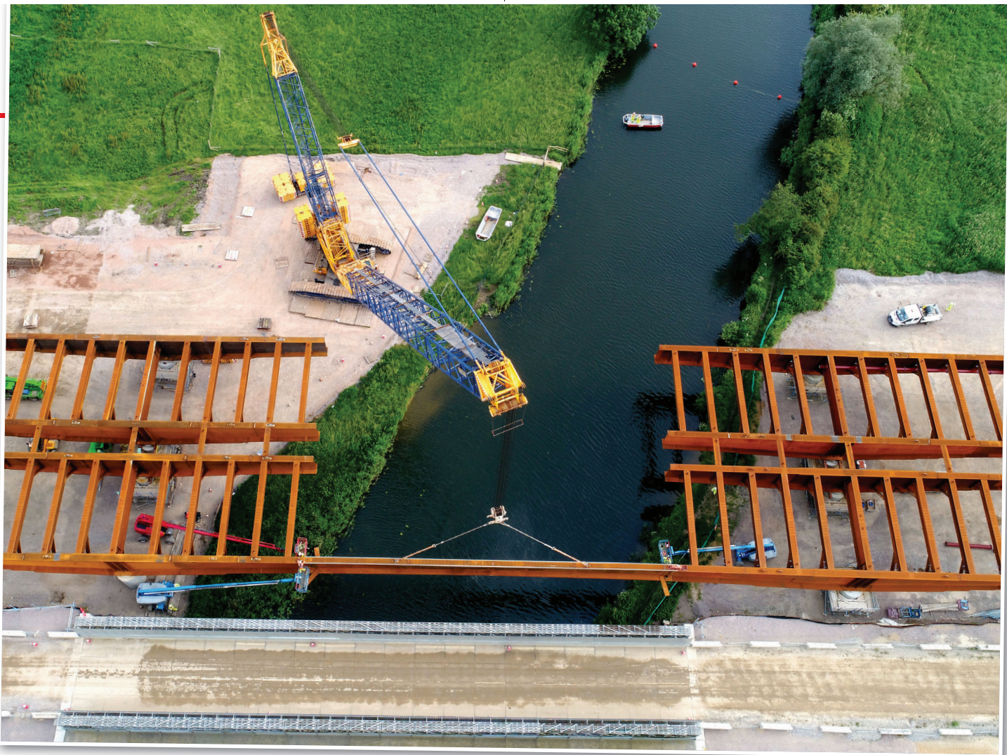
A 600 tonne crane places the first beam across the river near Buckden. Photo courtesy of Cleveland Bridge.
